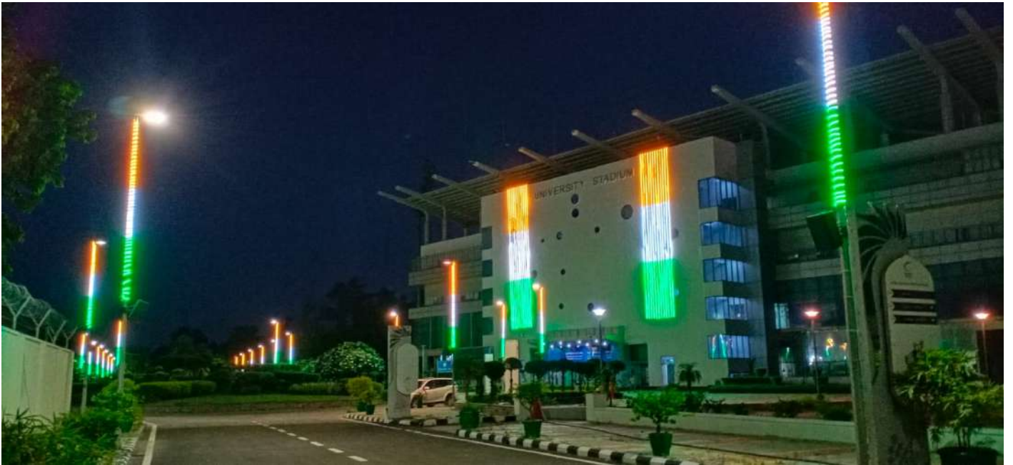
Cluster Innovation Centre Campus on the eve of 15 th August
